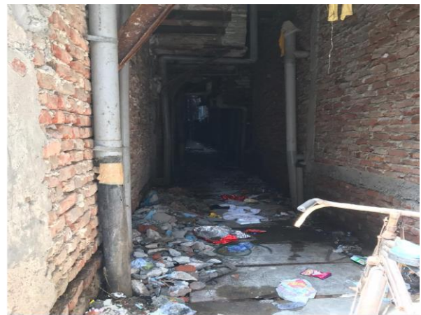
The toilet was built just along the drain line. Toilet pipelines from different houses directly connecting to the drain lines
