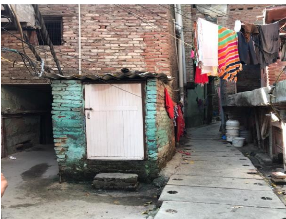
The toilet was built just along the drain line. Toilet pipelines from different houses directly connecting to the drain lines
